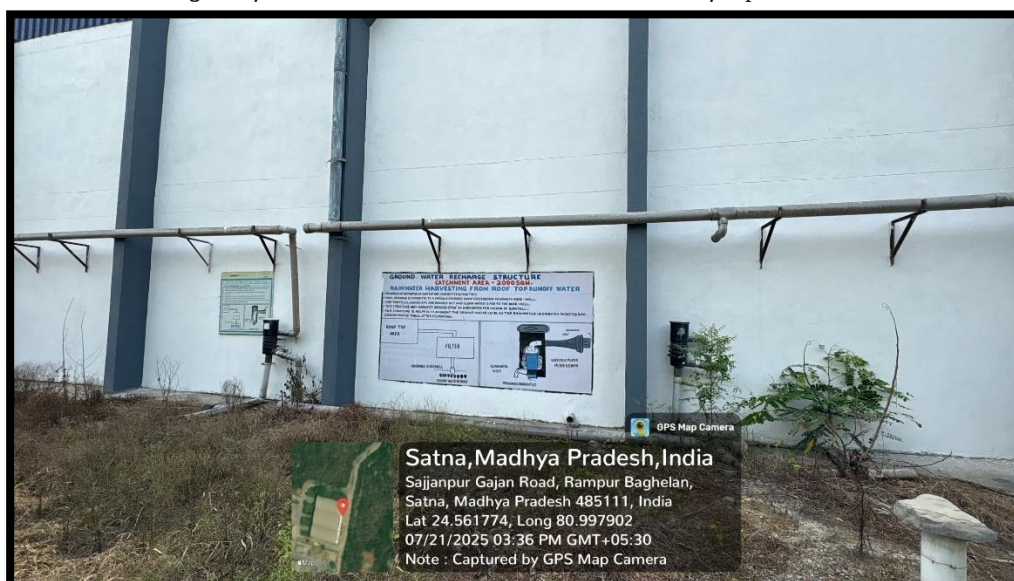
Roof Top structure
